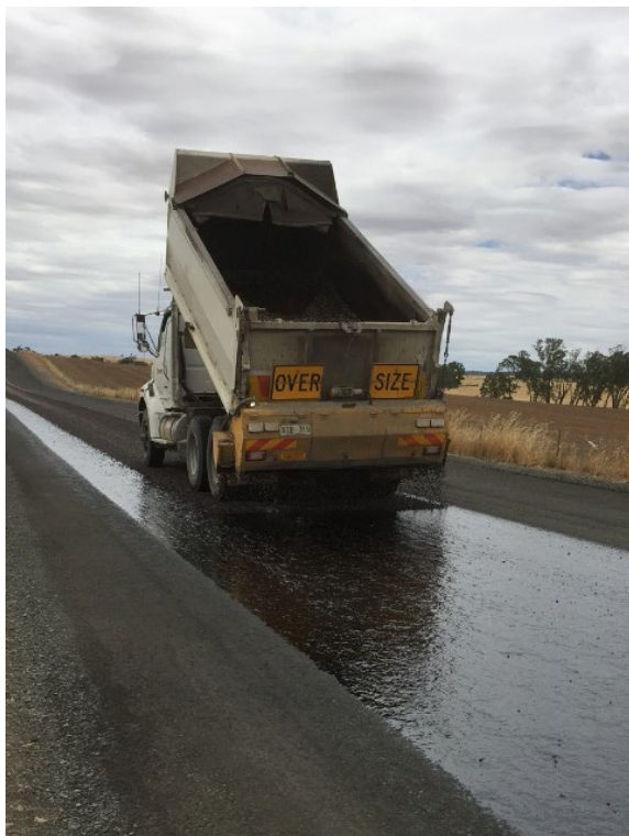
Sealing of Main Road 45
