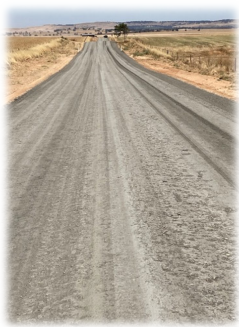
Bruce Hill Road – re-sheet
