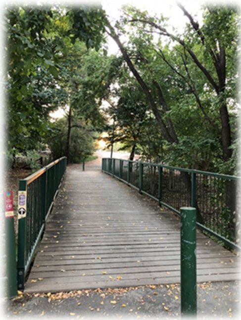
Centennial Park Bridge Auburn
