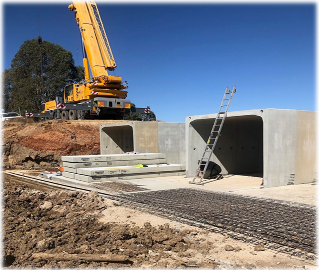
Harvey Highway Bridge Construction
